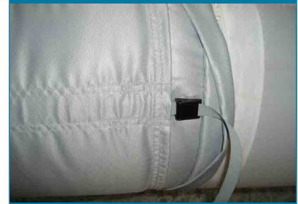
Close-up view of the tie belt
